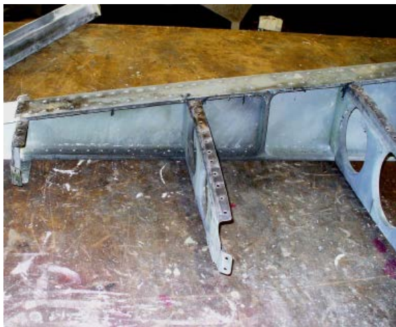
Pylon before repair...
