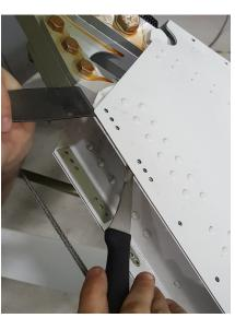
Remove rivet heads and aluminum chips between the skin and the channel
