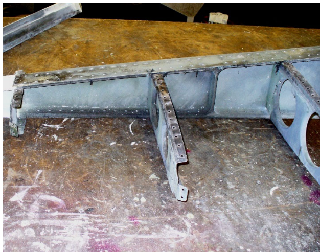
Pylon before repair
