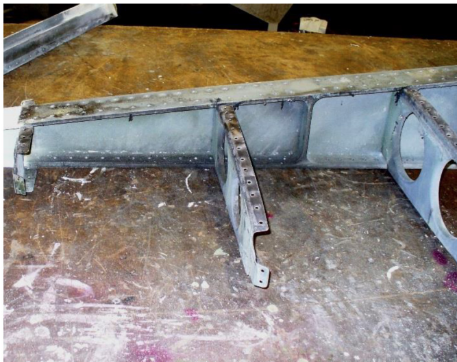
Pylon before repair
