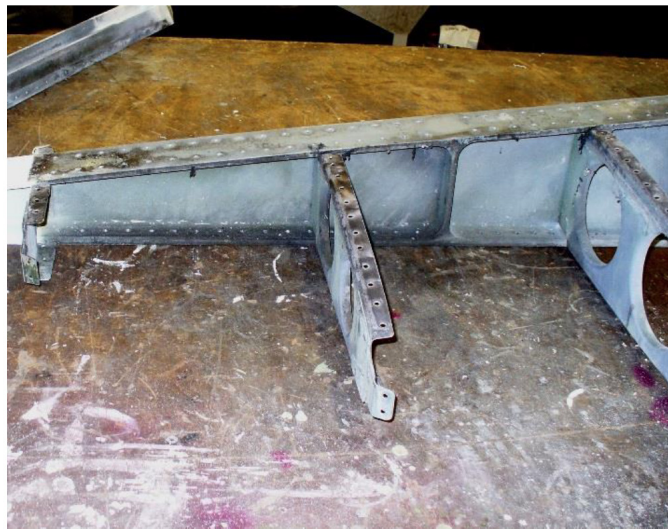
Pylon before repair
