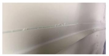
Condition 2 - Corrosion is visible around the stiffener, and the stiffener will need to be removed for further inspection and repair
