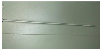
Method B - Corrosion is visible around and/or under the stiffener. The stiffener will need to be removed for replacement.
