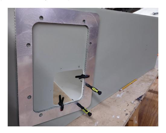
3b. Use clamps to hold the 1012335 template in position. This template will be lined up with the edges of the existing access hole. The small oval shaped hole should face in the most outward position. Mark the inside edge of the oval template.
